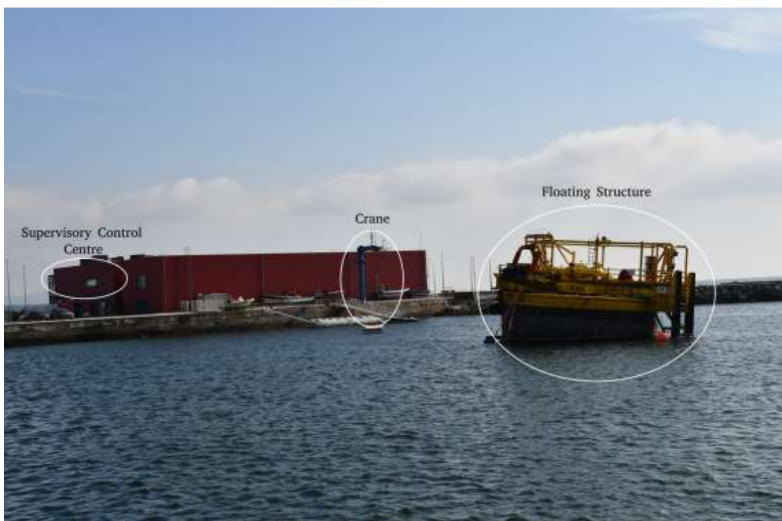
Figure 7 - ATLANTIS Test Centre Coastal Testbed and related infrastructures
